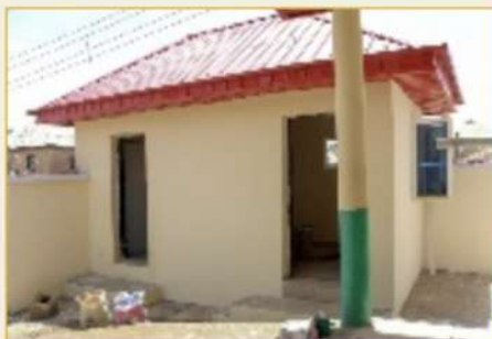
Health infrastructure under construction – expanding access to primary care at the grassroots.
